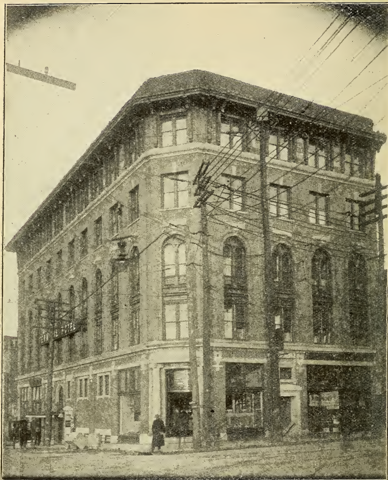
TERMINAL HOTEL Opposite Terminal Station
